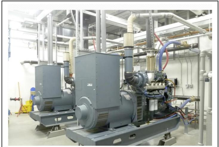
**Two 350 kW Detroit Diesel engine gensets (above) were removed from the old powerhouse, remanufactured and “marinized” (cooling system modified for water heating).**
